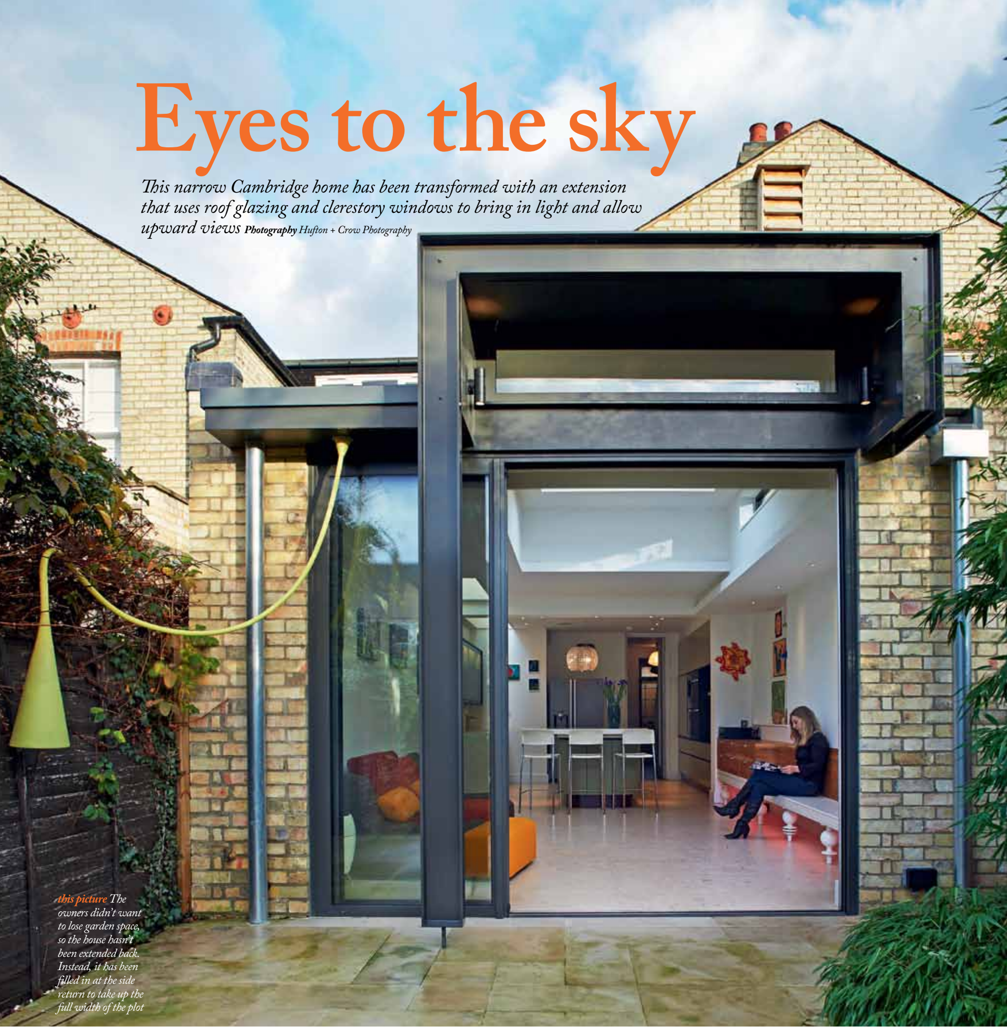
this picture The kitchen-living area is a long space (10x4.8 metres), so it was important to bring light into the heart of the building with roof lights and clerestory windows
